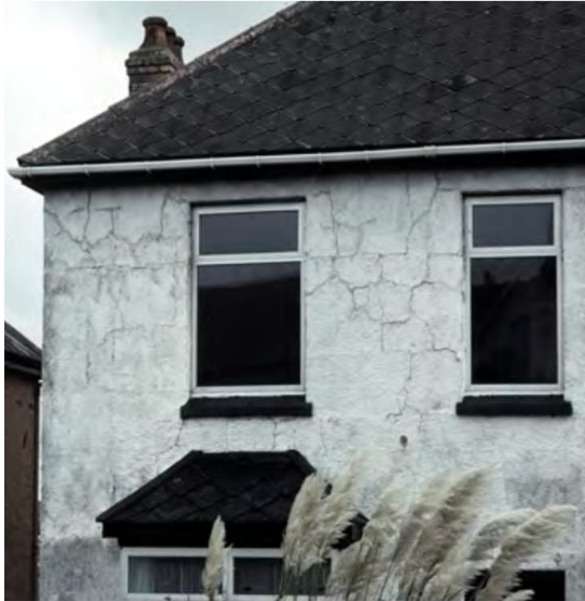
Figure 2 – Typical Mundic damage in residential building in South-West England [12].
