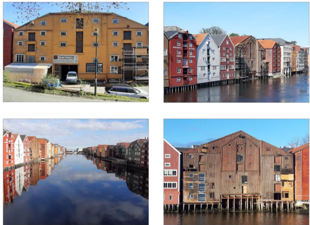
Figure 3. Views of Huitfeldtbrygga in Trondheim, Norway (personal images by the Authors).
