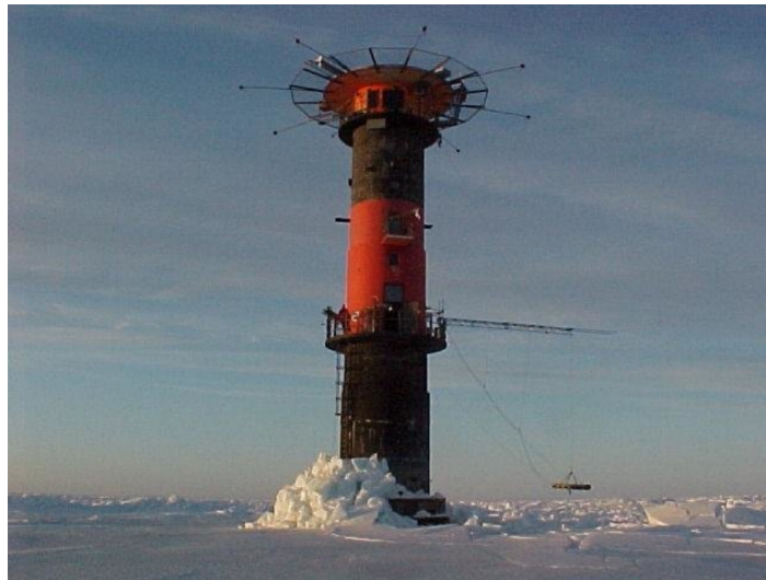
Figure 4-1: Photograph of the Norströmsgrund Lighthouse with a rubble pile after crushing failure of drifting level ice (Photo by Kari Kolari, VTT).
