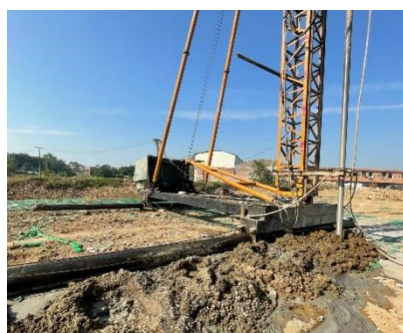
Figure 1. Deep mixing pile machine used in this study.
