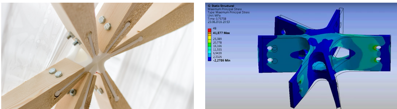
Figure 1. The node at the Printshell project and the ANSYS analysis at the project.
