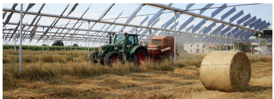
Figure 16. View of the dual use of land with the PV track system on the upper layer and agricultural works at ground level (photo: © REM).
