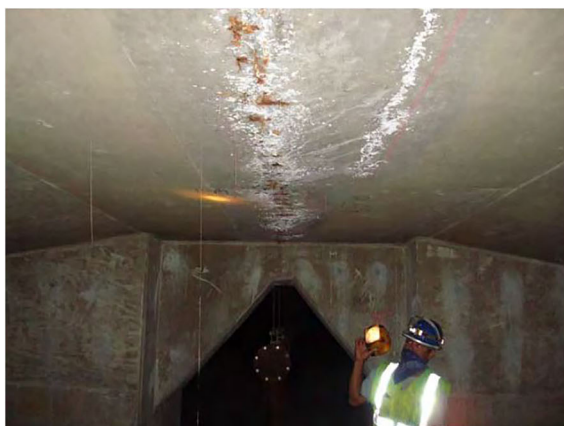
FIGURE 14 Warning signs detected in a posttensioned bridge in the Midwest of the USA. 29 Presence of efflorescence, delamination, and spall observed on a posttensioned box girder (left side). Voids and rust at different sections of the tendon (right side)
