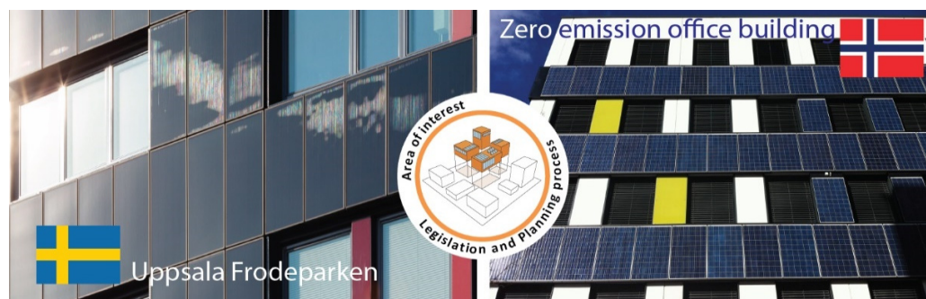
Figure 10. View of the building integrated photovoltaic facade in Uppsala Frodeparken (on the left. Source: © White Arkitekter) and in the Zero-Emission Office Building in Trondheim (on the right. Source: © Carmel Margaret Lindkvist).
