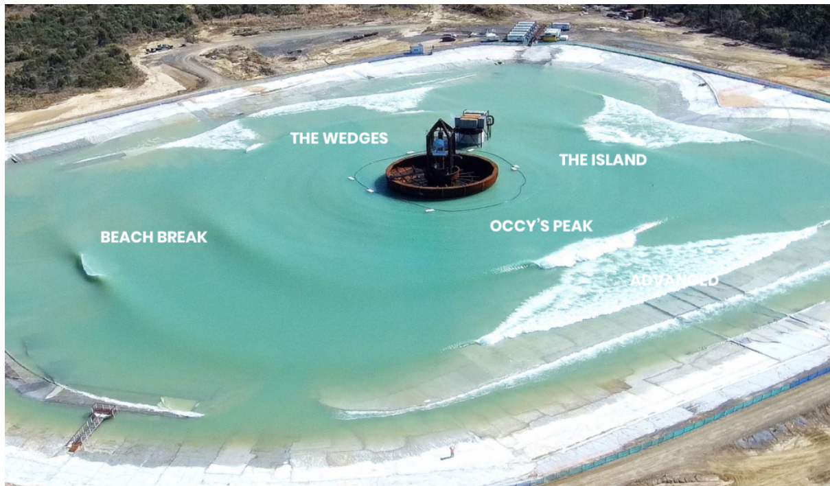
Figure 3.7: Photo of a artificial surf lake in Queensland (SurfLakes, 2020)
