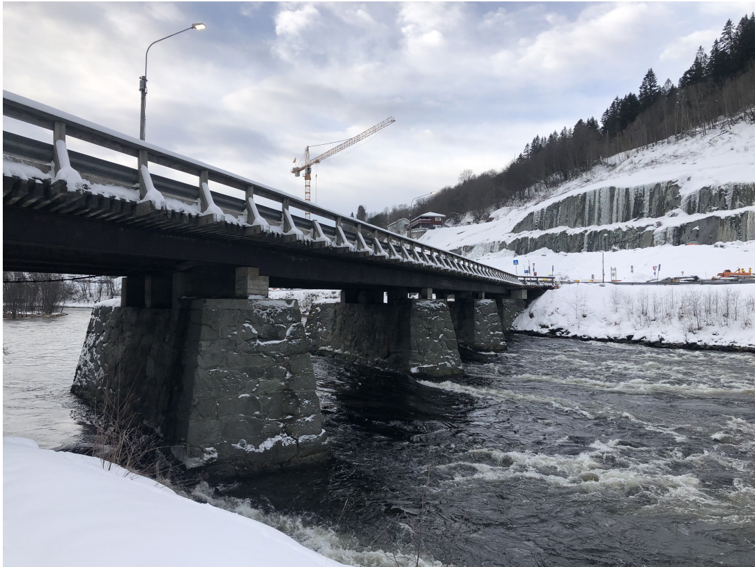
Figure 3.12: Downstream Sluppen bridge, taken 23. February 2022.
