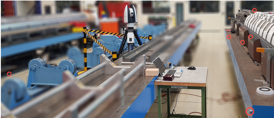
Figure 5.2: The setup of the LEICA AT930 laser tracker system used for the fiducialization of the higher-order corrector package. The tracker is mounted on a tripod in the center of the figure, the workstation is shown, and the targets used for re-orienting the tracker is highlighted by red circles.
