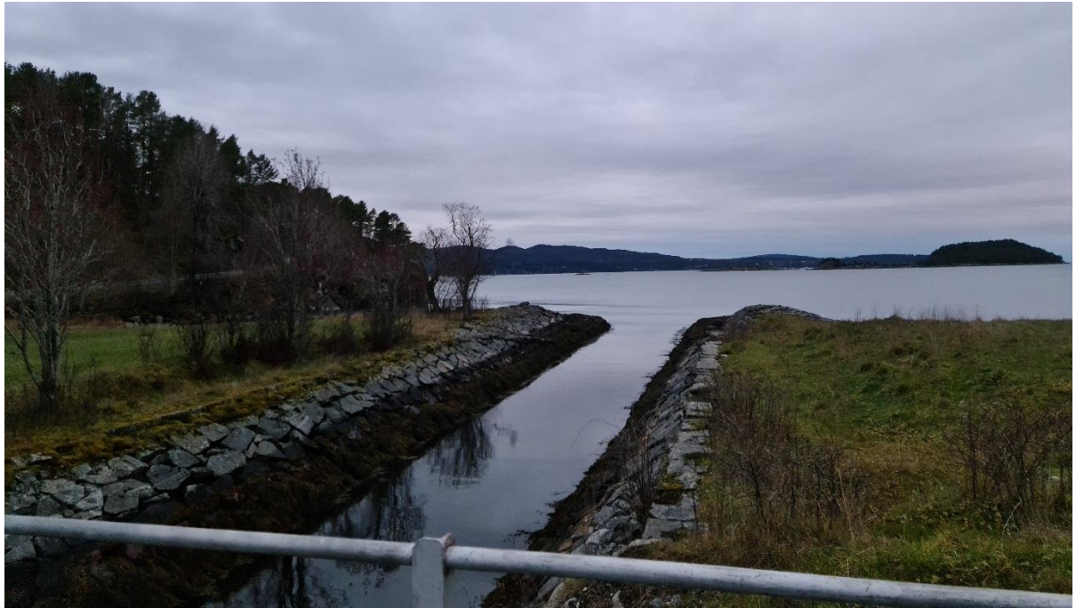
Figure 1.4 Nålundet (direction Freifjorden), the northern human-made inlet across the previously narrow isthmus. This channel allowed for water exchange between the outer fjordsystem of Freifjorden and Karihavet. Photo: Malin Bø Nevstad, 2022.
