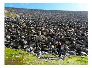
**Figure 1.** Placed riprap constructed on the downstream slope of Oddatjørn dam, a 142 m high rockfill dam built in Suldal, Norway [2].
