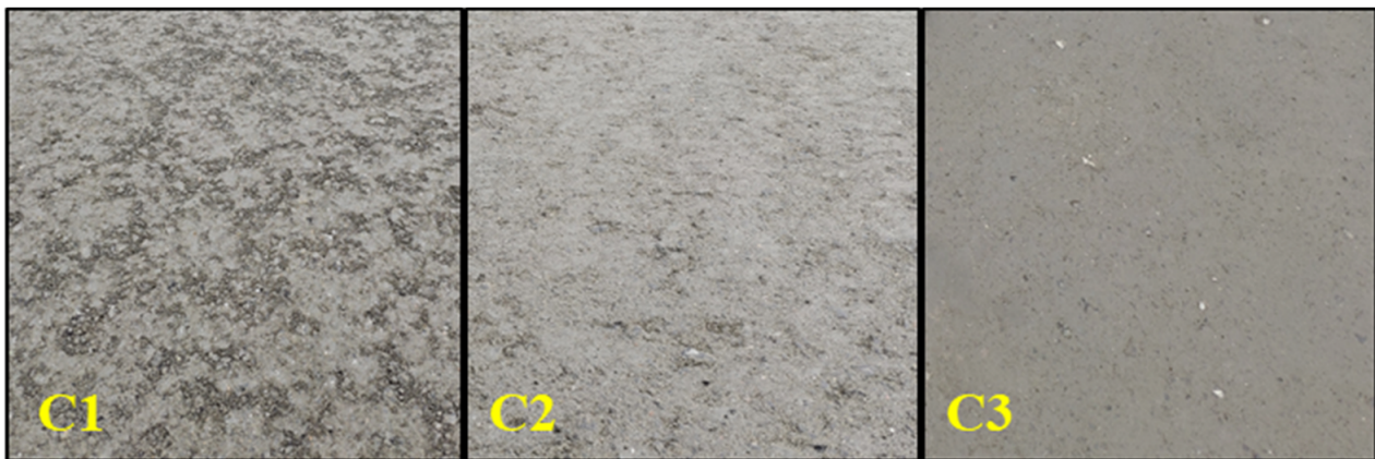
Figure 6. Surface of base layer compacted according to the C1–C3.
