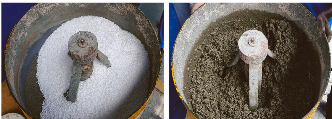
Fig. 3. The mixing of EPS lightweight aggregate concrete.
