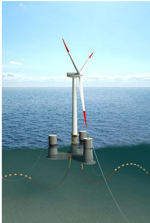
Figure 1 The LIFES50+ OO-Star Wind Floater Semi 10MW structure [11].
