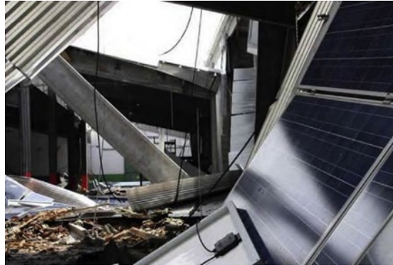
Figure 8. Collapse of an RC building, which received only energy retrofitting after the 2012 Emilia-Romagna earthquake.
