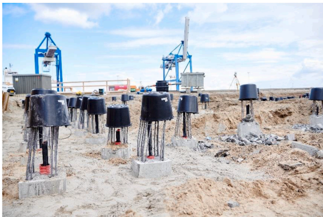
Fig. 6. Driven precast concrete quadratic energy piles with inner pipes; image courtesy: Centrum Pæle A/S [89].
