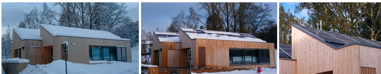
Fig. 2. ZEB Living Lab after a snowfall in late January 2015 (left); The snow cover sticks to the frame and slides off only partially after a snowfall in late November 2015 (middle); detail of the roof geometry with the tilted and flat parts, the weather station and the three rows of modules installed and the lowest part free from the PV modules (right). Photo credit: Clara Good.
