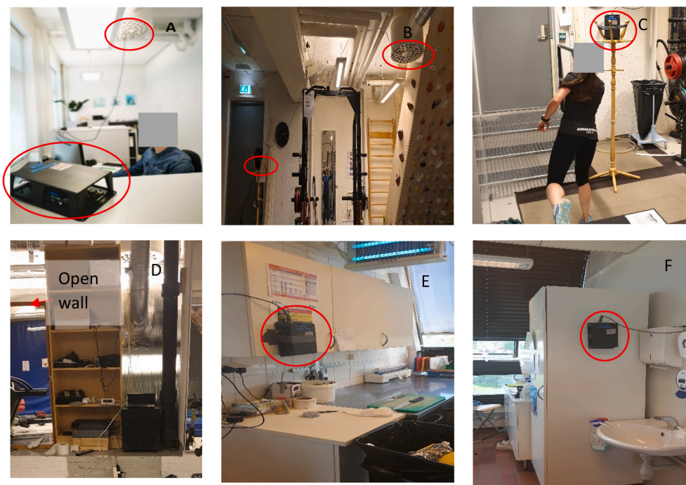
Fig. 3. Installations of measurement equipment: (A) in the office; (B), (C) and (D): in the gym; (E) in the kitchen; (F) in the canteen.
