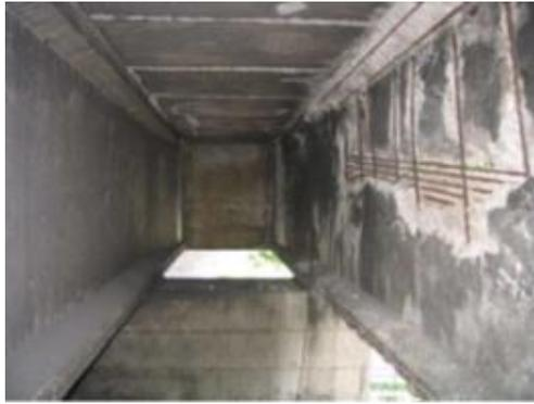
**Figure 3.1.19.** Annone Overpass (ID-21). Damage observed on internal surfaces of the prefabricated beams in 2006 (Di Prisco et al, 2018).
