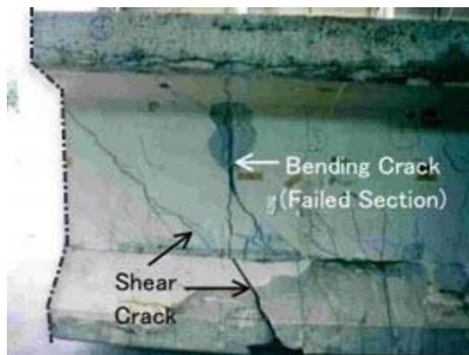
**Figure 3.3.5.** Kure-tsubo Bridge (ID-39). Cracks around failed section of beam S3 (Tanaka et al, 2001).
