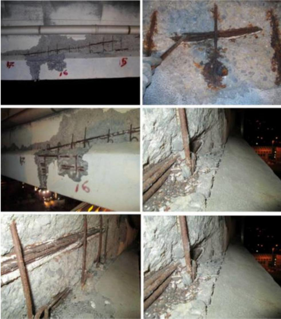
**ID-6.7.** View of cables toward the support in 2011 (top) and 2013 (middle). Zoom of the cables in 2013 (bottom) where corrosion and partial pitting can be appreciated (Nutti et al, 2020).
