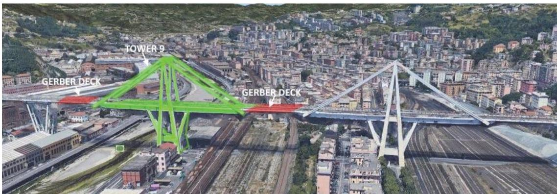
**Figure 6.3.** Involved structure in the collapse: tower and Gerber decks (Bazzucchi et al, 2018).
