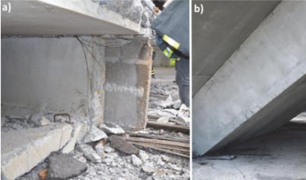
**ID-5.4.** Prestressing cables in the collapsed joint area (a); external concrete conditions (b) (Bazzucchi et al, 2018).
