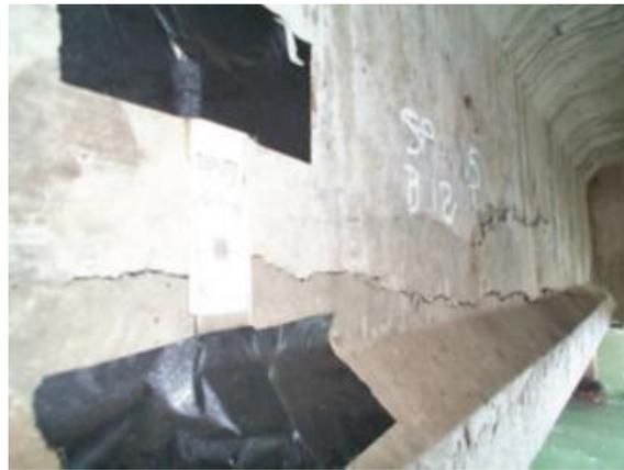
**ID-3.2.** Typical longitudinal web cracking along a beam (Papè and Melchers, 2011).
