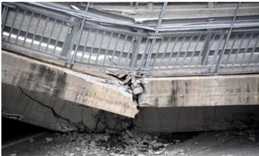
**ID-5.2.** Bridge beam: mid span fracture
