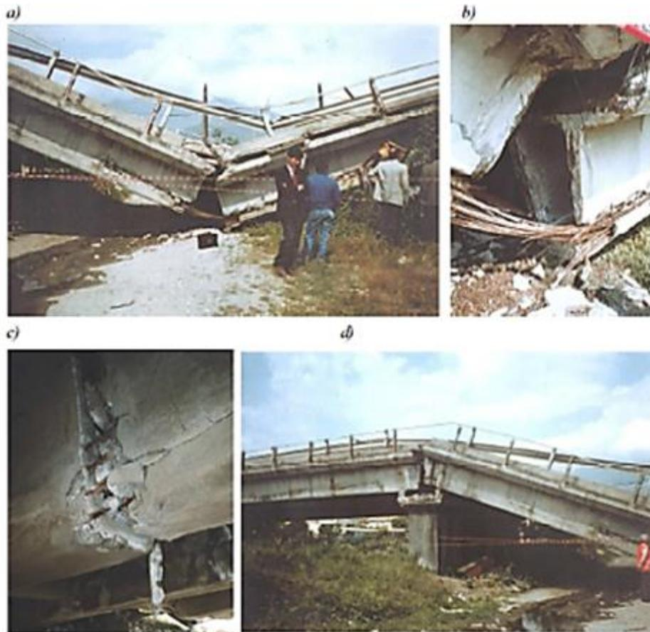
**ID-2.3.** S. Stefano Viaduct: a) collapse of the viaduct; b) slippage of cables; c) opening of joints; and d) rotation of the deck (Colajanni et al, 2016).
