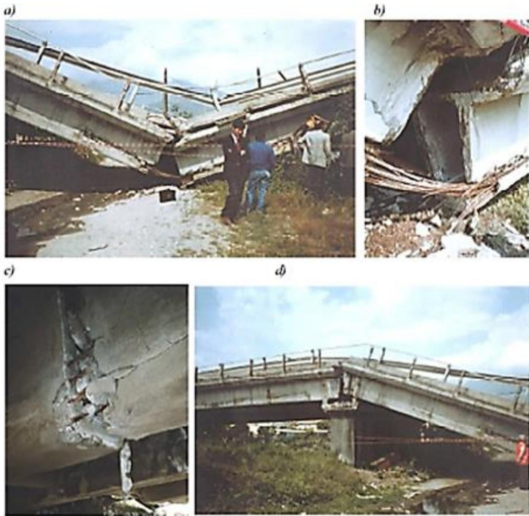
**Figure 3.3.4.** S. Stefano Viaduct (ID-2): a) collapse of the viaduct; b) slippage of cables; c) opening of joints; and d) rotation of the deck (Colajanni et al, 2016).
