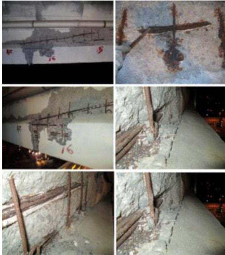
**Figure 3.1.18.** Polcevera Bridge (ID-6). View of cables toward the support in 2011 (top) and 2013 (middle). Zoom of the cables in 2013 (bottom) where corrosion and partial pitting can be observed (Nutti et al, 2020).
