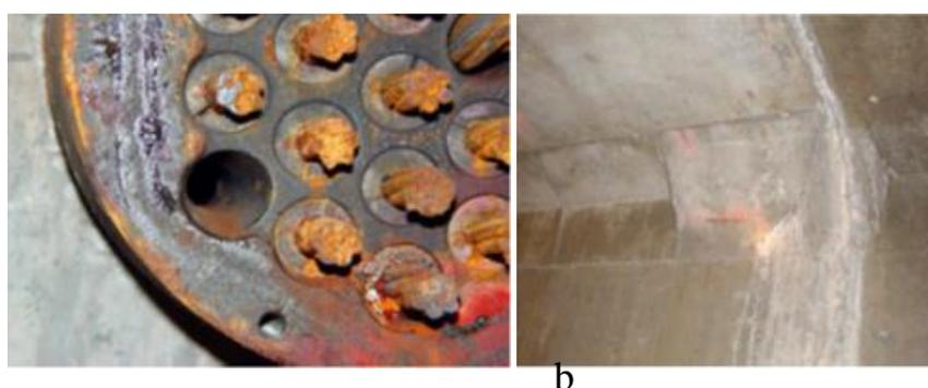
**Figure 3.1.10.** San Francisco – Oakland Bay Bridge (ID-14): a) close-up view of an anchorage head showing signs of corrosion from water collected at the anchorage; b) view of a crack at an anchor block showing efflorescence (Reis, 2007).
