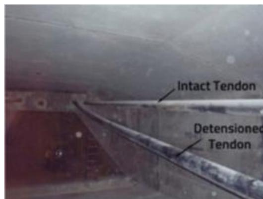
**Figure 3.3.7.** Ringling Causeway Bridge (ID-15). Detensioned tendon discovered in July 2011 (Ahern et al, 2018).
