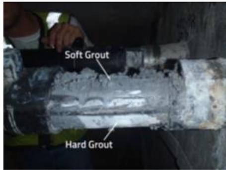
**Figure 4.2.2.1.** Segregation of the grout material observed near the high points of the tendon profile in Ringling Causeway Bridge (ID-15) (Ahern et al, 2018).
