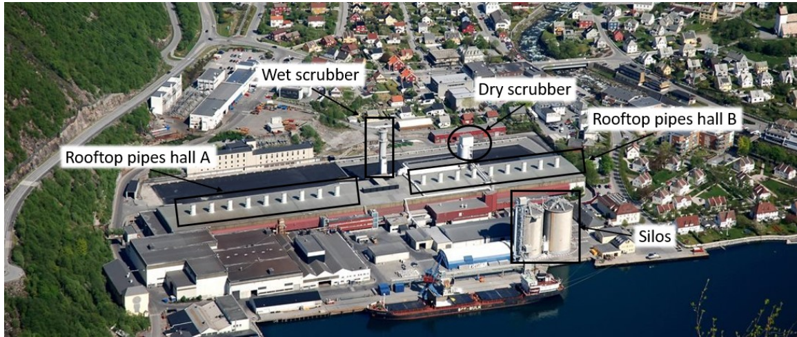
Figure 3.1.2: Close-up picture of Hydro Aluminium Høyanger [9]. The figure includes the placement of the rooftop pipes of hall A and B, the wet- and dry scrubber and the silos.
