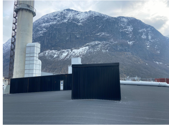
Figure 3.1.8: East side of the plant.
