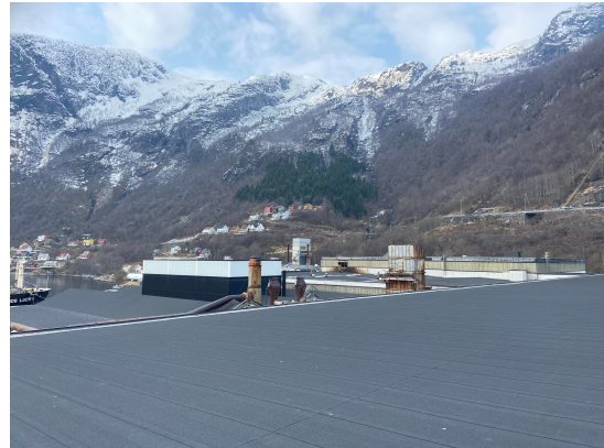
Figure 3.1.10: South-west side of the plant.
