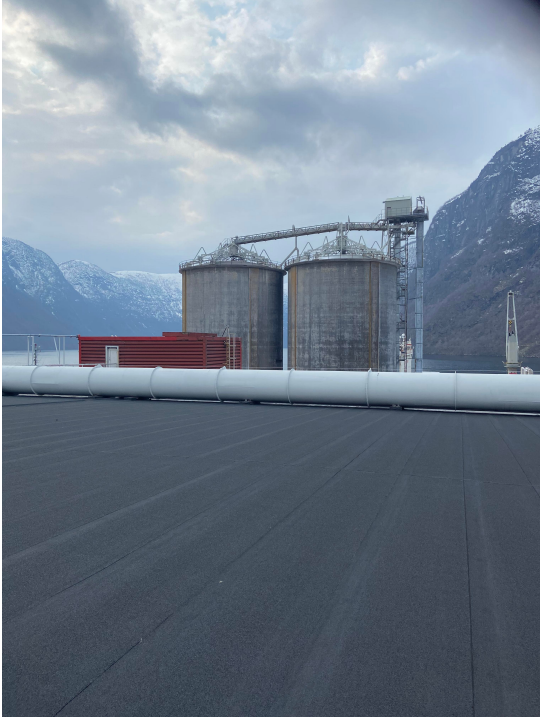
Figure 3.1.4: Silos at Hydro Aluminium Høyanger.
