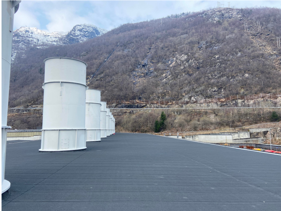
Figure 3.1.11: West side of the plant.
