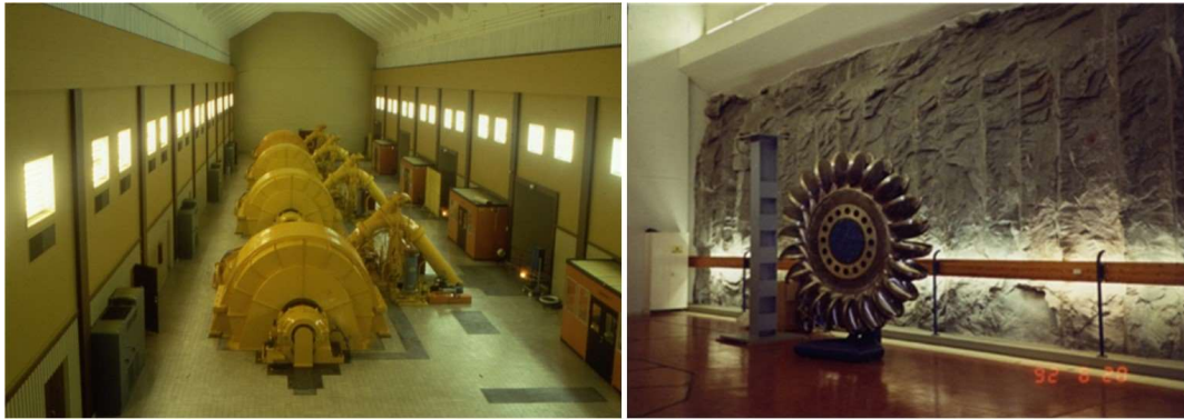
Figure 4: The Aura underground hydropower station, commissioned in 1952 (left) and Tafjord K-5 underground powerhouse station commissioned around 1970s (right)
