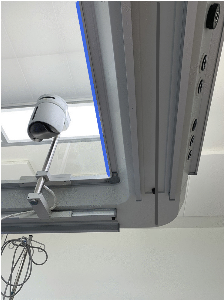
Figure 16: Picture showing the inside of the LAF canopy in blue and center of the LAF canopy in dark grey
