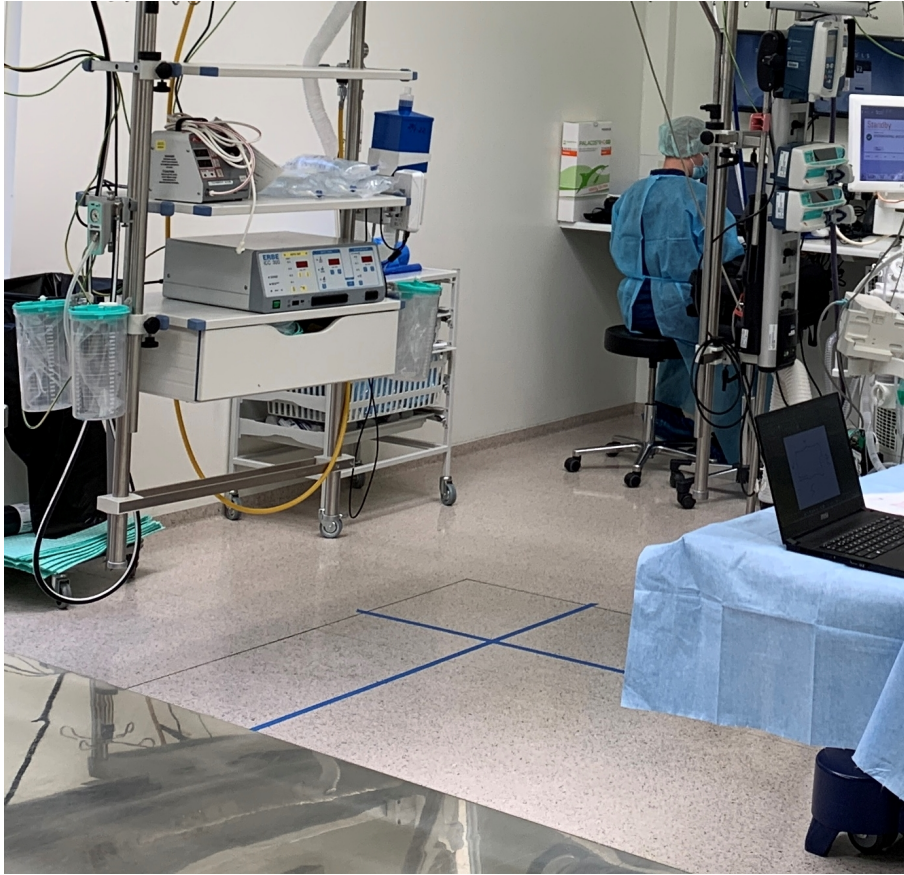
Figure 15: Picture showing the grey floor marking indicating the center of the LAF canopy and the blue tape indicating the inside of the LAF canopy
