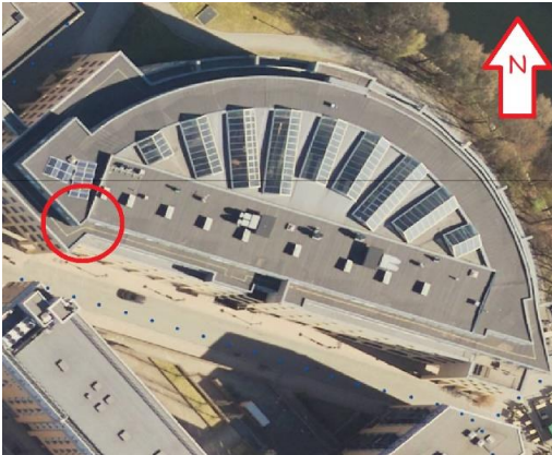
Fig. 2. Situation plan for the building at Norconsult Headquarters in Sandvika (59°.53'N, 10°.31'E), Norway, where full-scale test office is situated on the top (6 th ) floor
