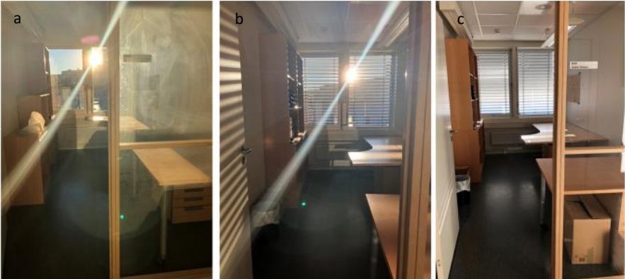
Figure 3 Typical office with windows oriented against south or west, a) excessive low-angled sunlight brings discomfort to the users of an office space; b) the sun-shading device is closed and adjusted to protect visual comfort and enable daylight; c) the sun shading slats are completely closed to ensure the visual comfort of the office user.
