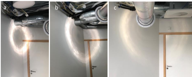
Figure 35 Circular belt formed by light output from the HLP with clear transparent diffuser on the adjacent wall (2 m-distance). a) in January at noon; b) in March around 11AM; c) in March around 2PM;
