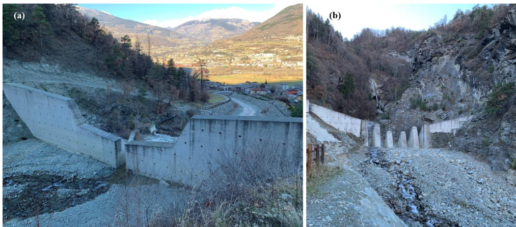
Figure 2.9 Examples of rigid barriers in Aosta Valley (Italian Alps) (a) Closed rigid barrier; (b) Slit sectional barrier
