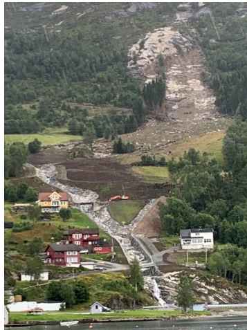
Mitigation measures for a debris flow in Jølster, Norway
