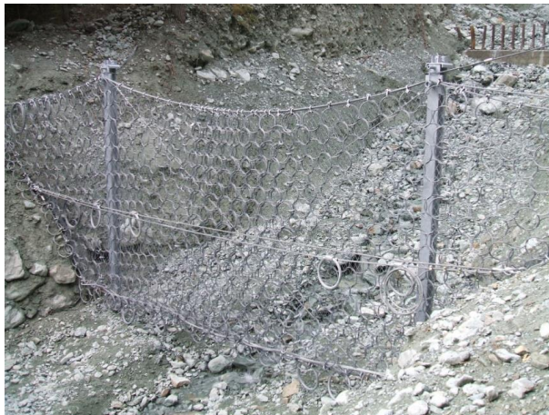
Flexible barrier installed in the field
