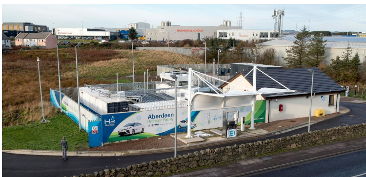
Figure 2.1: Hydrogen production and refueling station in the city of Aberdeen, Scotland
