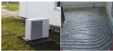
Figure 3: Heat pump and the underfloor heating system
