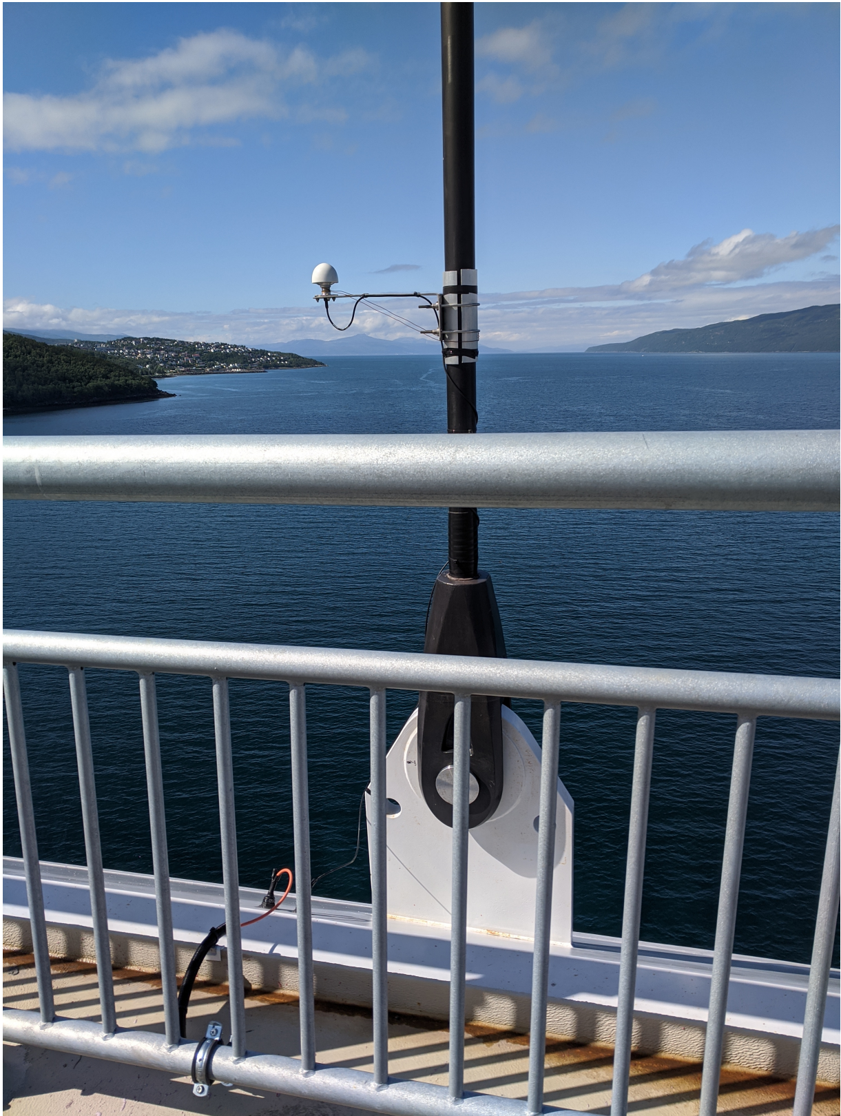
Figure A.3: Connection of the hangers to the bridge deck, with equivalent connections to the main cables.
