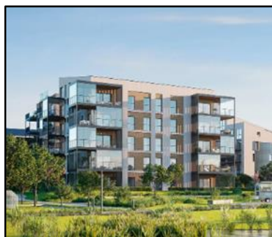
Figure 3-2 The selected apartment building- Typology: Verket Panorama
