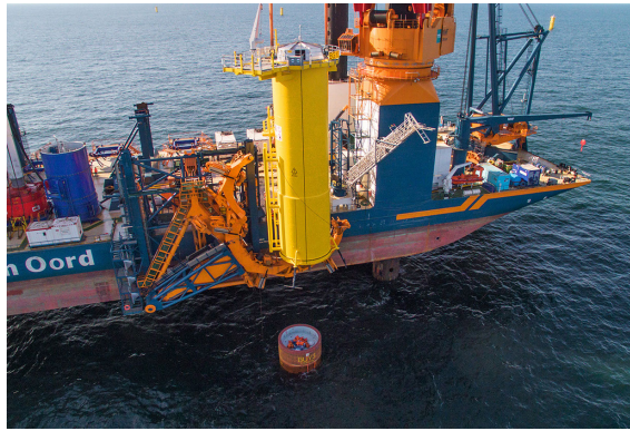
Figure 6: The installation of a transition piece on a monopile.
