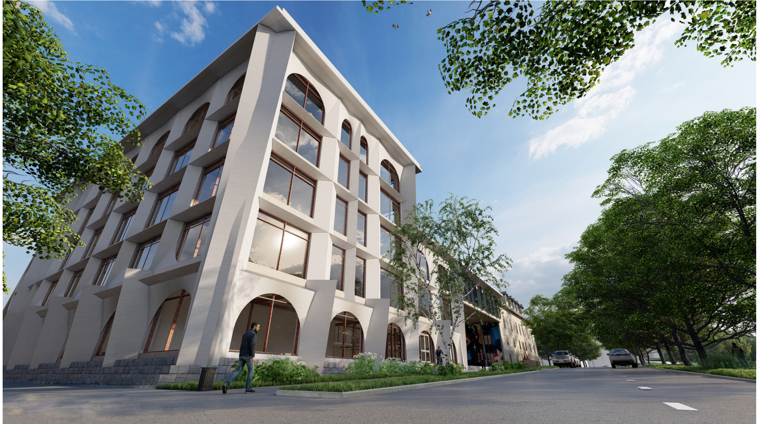
View from western approach on Høgskoleveien of southern facade
