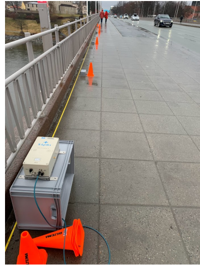
(b) Sensors and main unit on upstream measurement.
