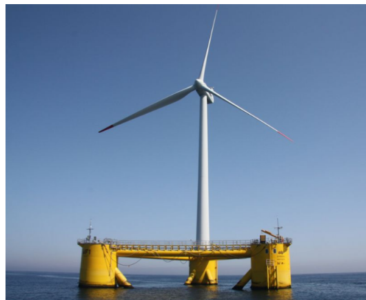
Figure 2.2: One of the semi-submersible wind turbines installed in the Kincardine Offshore Wind project [10].
