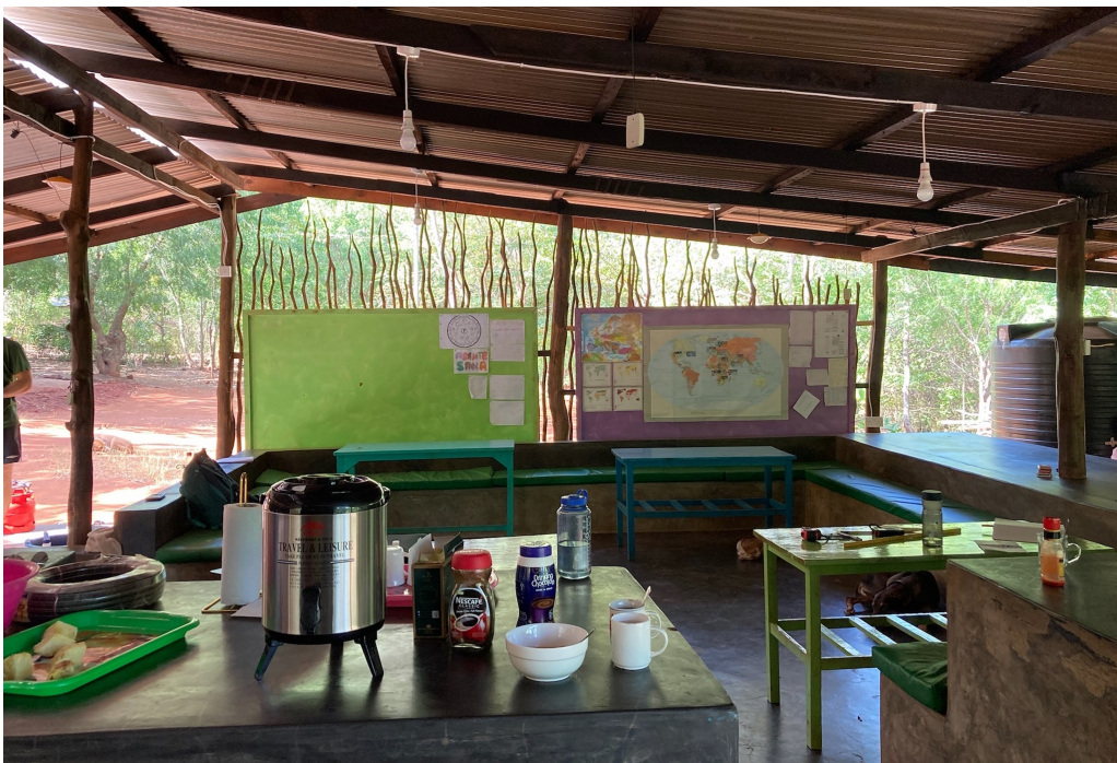
Figure 22: Inside of kitchen.
