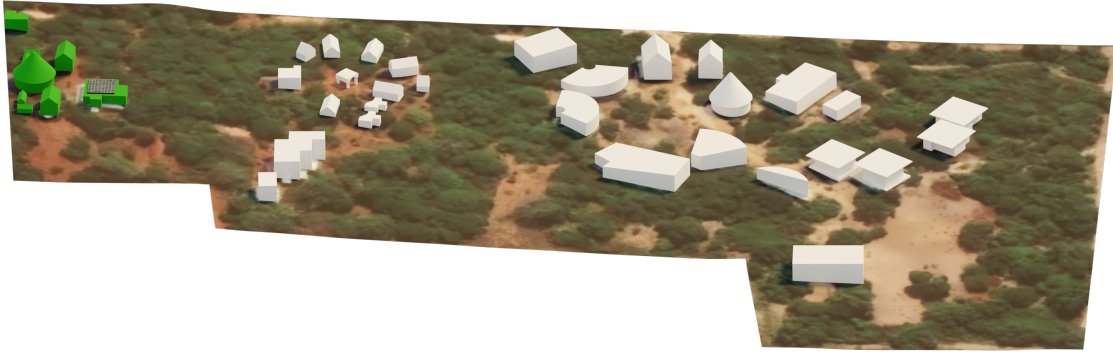
Figure 55: Cluster 1 in green with PV panels on kitchen.
