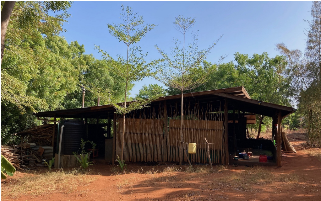
Figure 21: Outside of kitchen.
