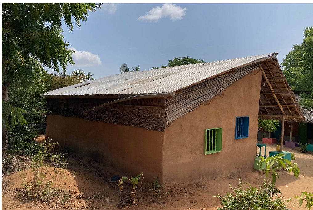
Figure 27: Outside Staff Room.
