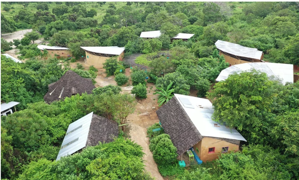
Figure 5: Drone picture of parts of the property.
