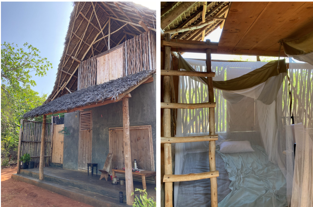
Figure 30: Outside and inside sleeping area main hut.
