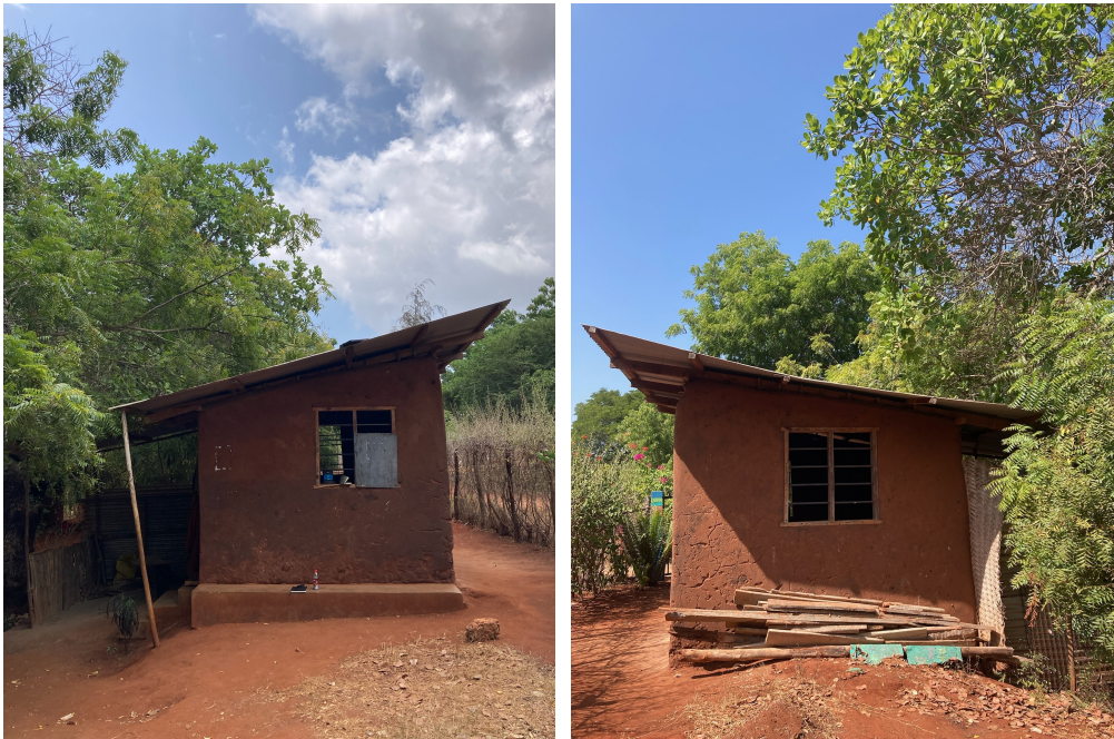
Figure 28: Side views of security building.
