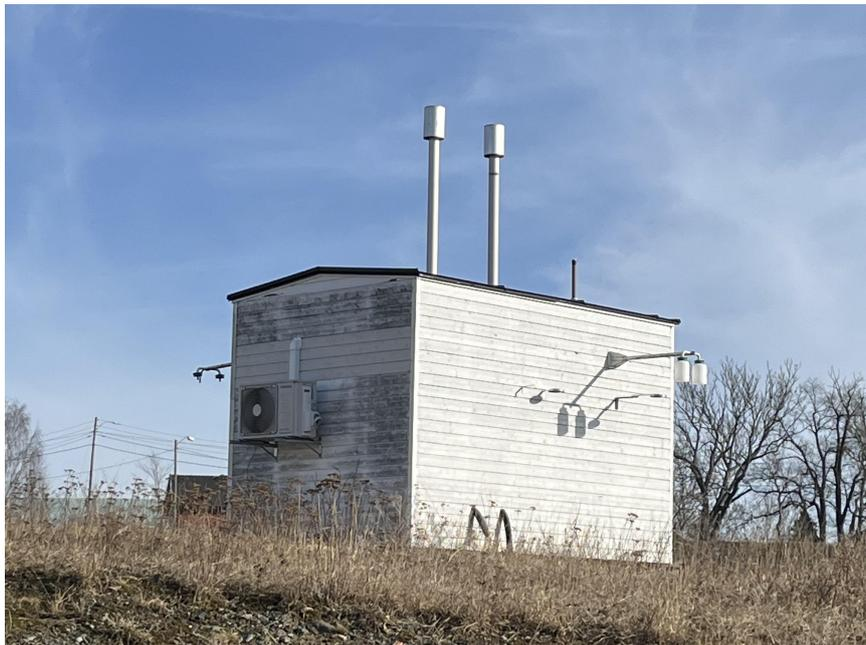
**Figure 3.1:** An air monitoring station at one of the visited sites. The station sends live data to the institute database. Additionally, samples for analysis are regularly collected at the station. *Picture is taken with permission from the participant showing us around during an observation visit.*
