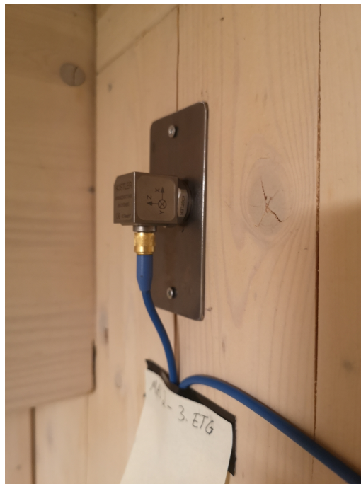
Figure 4.6: Accelerometer installed on a CLT wall
