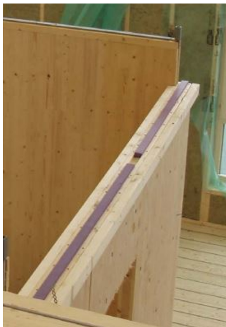
Figure 2.3: Vibration-damping intermediate layer. Photo: [15]
