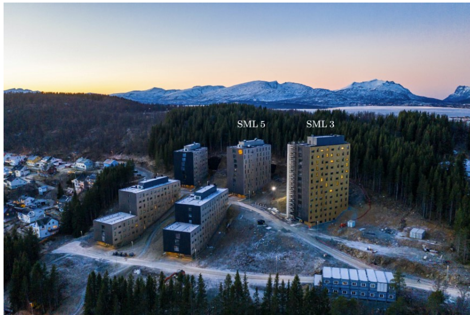
Figure 1.3: Dramsvegen Panorama student housing. The two buildings in question are located to the right [14].
