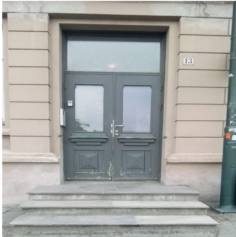
Figure 16: Main entrance of Elgesetergate 13 [Photo: by author]
