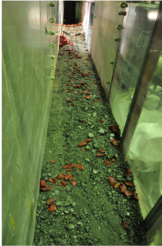
Figure 3.8: Riprap, shell, and filter material mixed after dam breach
