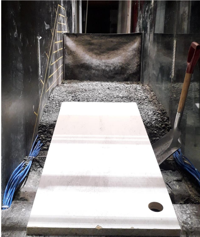
Figure 3.4: Dam with central core under construction
