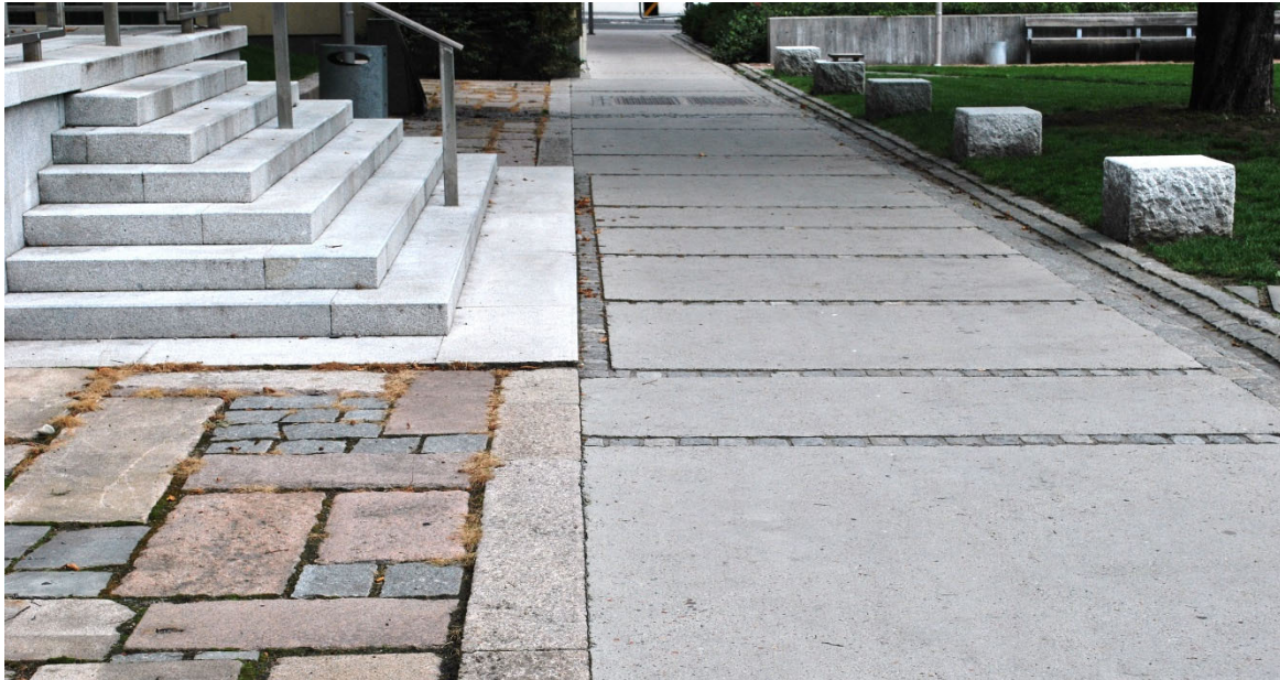
Figure 23 Reused granite and orthogonal slabs from demolished concrete used as outdoor ground covering in Pilestredet park, Oslo. (Photo: Helge Høifødt) 57
