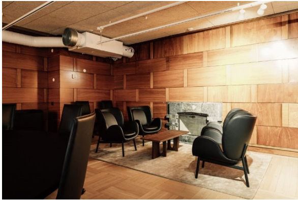
Figure 29 Interior wood paneling was reused to preserve some of the buildings unique character. 64
