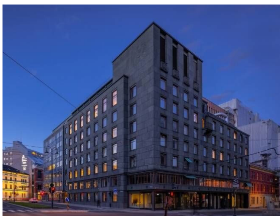
Figure 27 The exterior facade and windows were retained due to being listed for architectural preservation. 64
