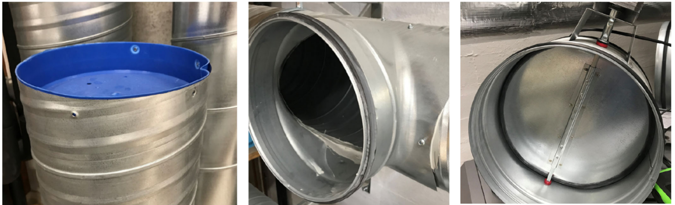
Figure 21 Round duct, duct parts and duct damper. Photo: SINTEF Community. Feil! Bokmerke er ikke definert.
