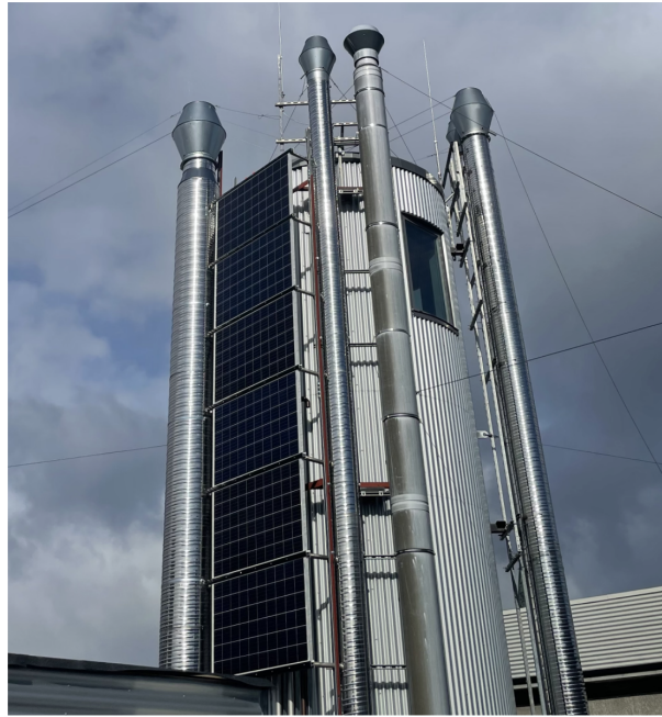
Figure 4.2: Placement of PV panels on the roof of the Thermal Laboratory on the fourth floor.
