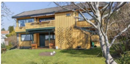
(a) The house in Kristiansand before renovation.
