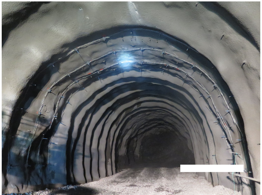
Ryfylke tunnel during construction. Photo: Ahmed Al-Samarray (NPRA)
