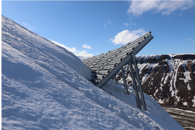
Figure 5.3: Sukkertoppen snow support structures
