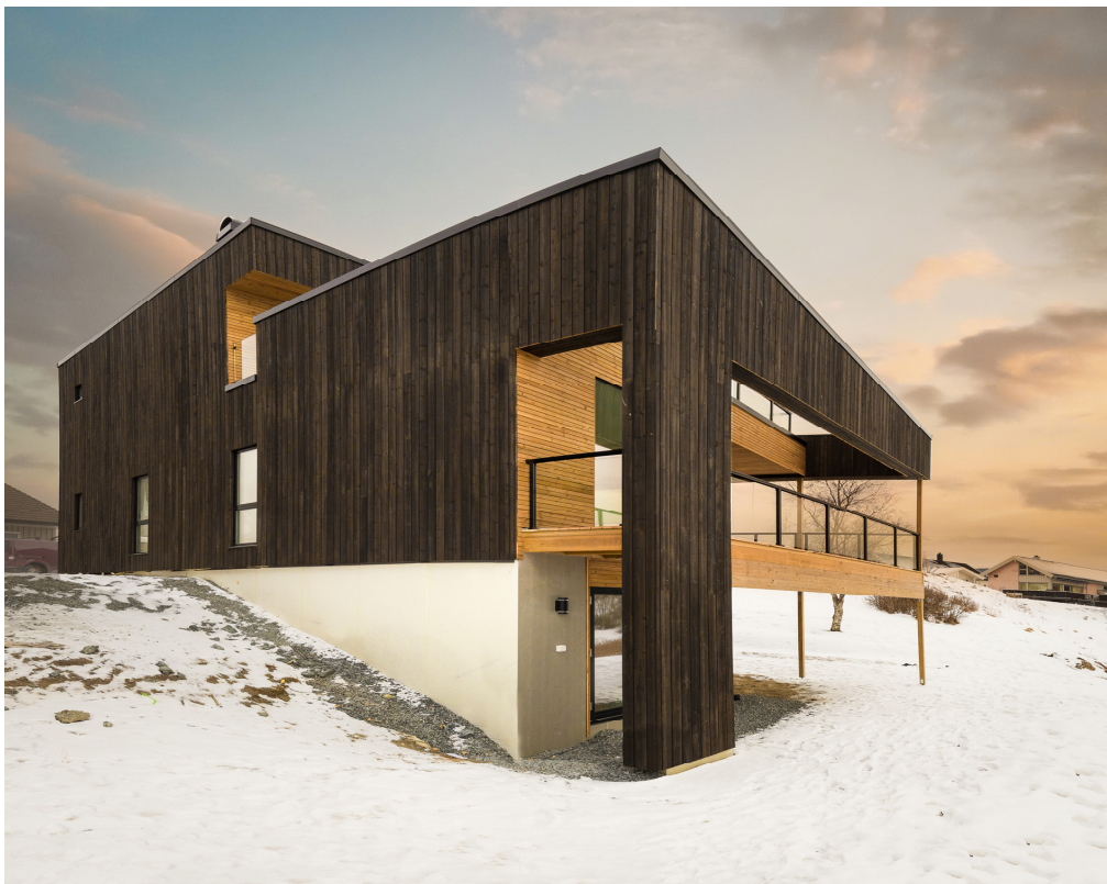
Figure 1. It is common for house manufacturers to supply houses with semi-basements on sloping plots. In this single-family dwelling, half of the exterior walls of the lower floor is below grade, and the rest has access to the outdoors. Bathrooms, laundry rooms, corridors, and technical rooms are often located in the rear part. It is common for bedrooms and living rooms to have one or more walls facing the terrain and at least one wall with windows. Fossen is a house model designed and manufactured by Norgeshus (Image: Norgeshus).
