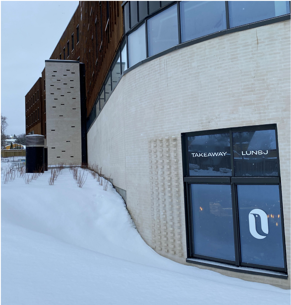
Figure 3. Multipurpose building with a restaurant located in the basement. A kitchen is located next to the below-grade exterior wall.
