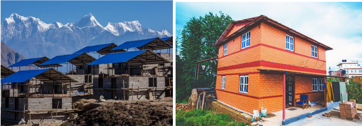
Figure 5-11 Houses built using CSEB, picture from Build up Nepal [69].
