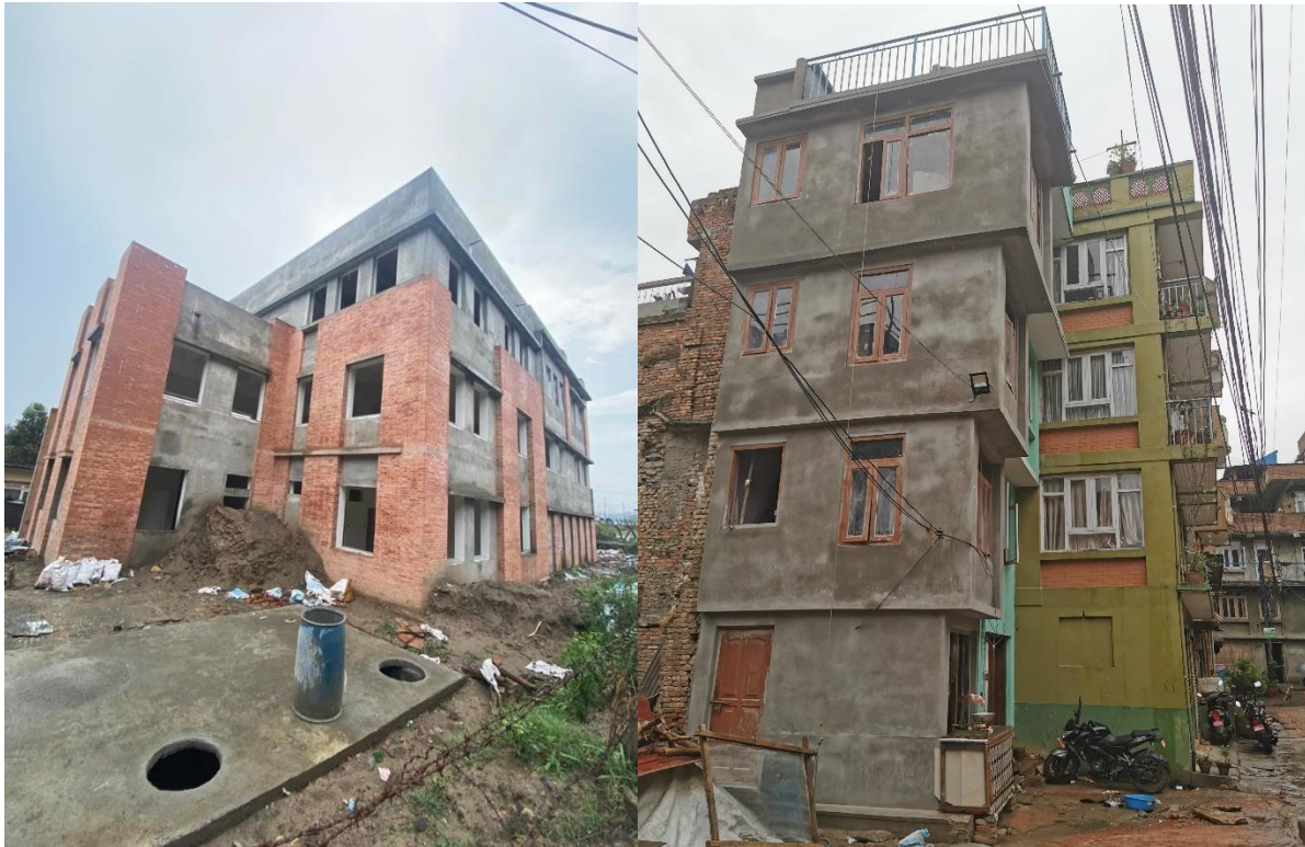
Figure 2-4 To the left, a new school building where concrete and red bricks are combined. Picture to the right shows a concrete building in Kirtipur. The first floor is used as a store, which is a typical set up for buildings in Nepal. (Pictures from field study)
