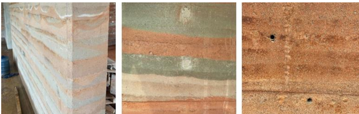
Figure 5-9 Different rammed earth walls.
