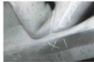
Chord or bracing localised buckling
