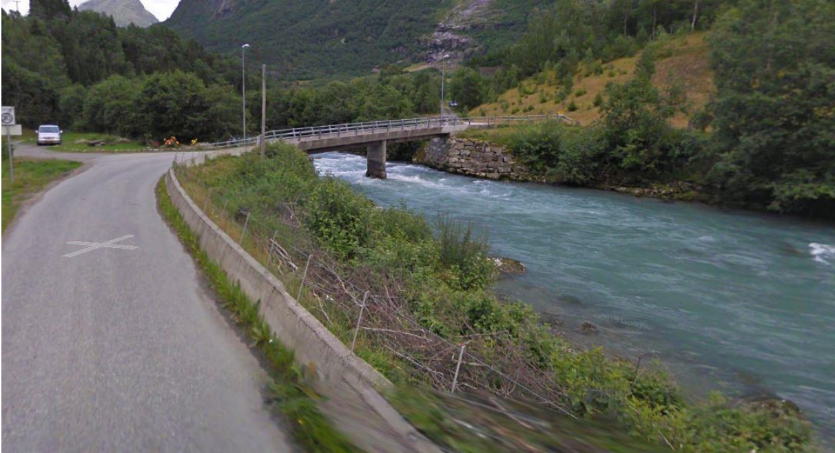
Figure 72: Hjelle bridge seen from the north side of the river.
