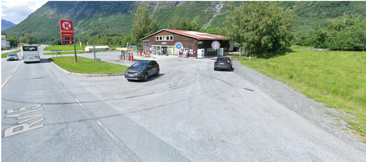
Figure 62: The petrol station and store, which was flooded in 1995. Picture captured from Google Street view.
