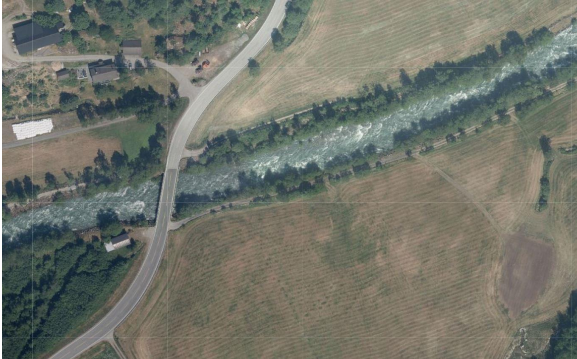
Figure 57: The first bridge after Videdøla turns into Hjelledøla, with a 2m GLOF. Captured from Norgebilder.no
